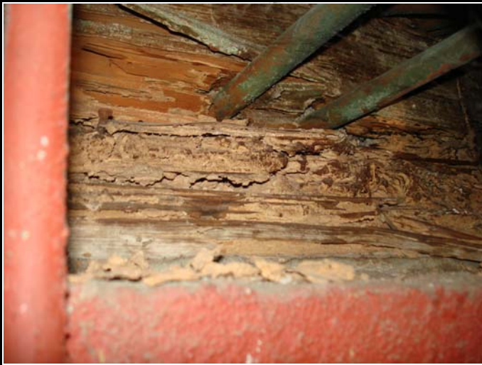
Damage to sill beam in basement.
