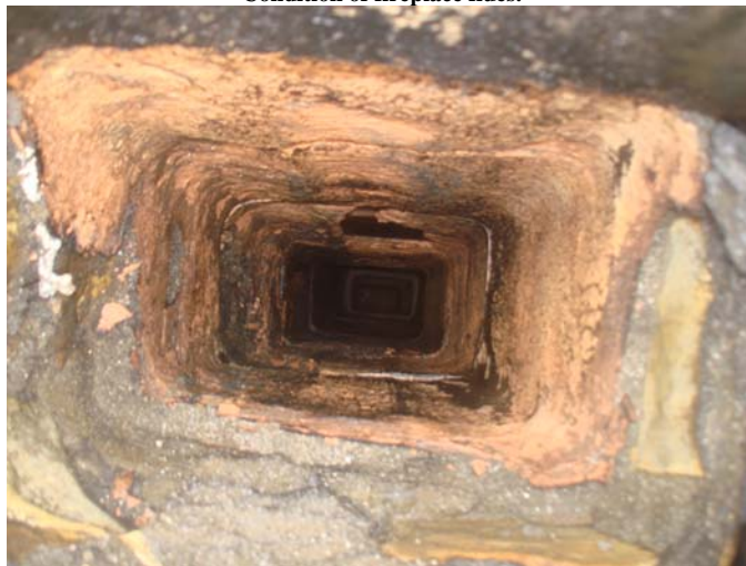
Condition of boiler flue.
