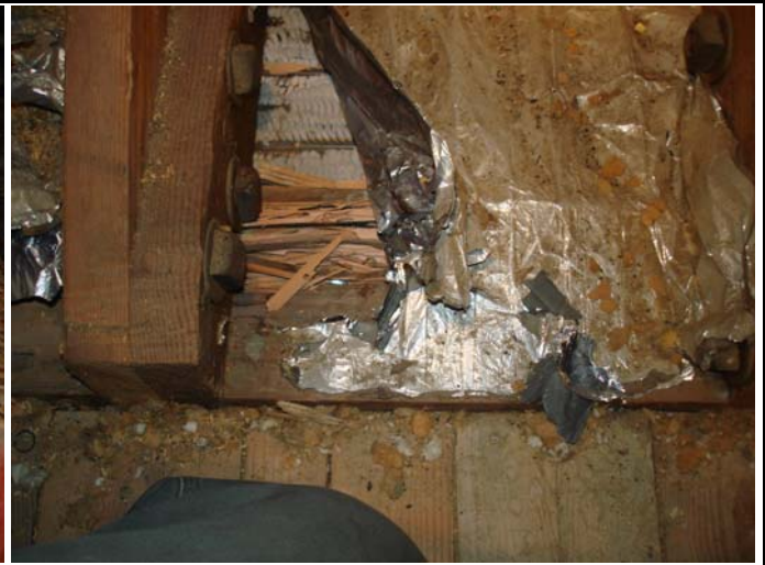
Damage to sill beam in basement.
