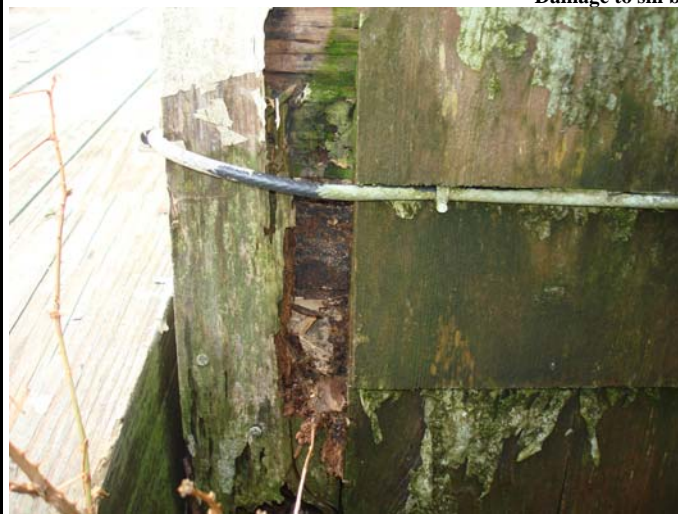
Termite damage & decay of the sill beam on the exterior.
