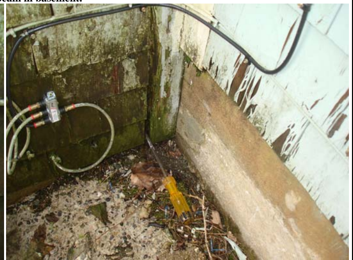
Termite damage & decay of the sill beam on the exterior.
